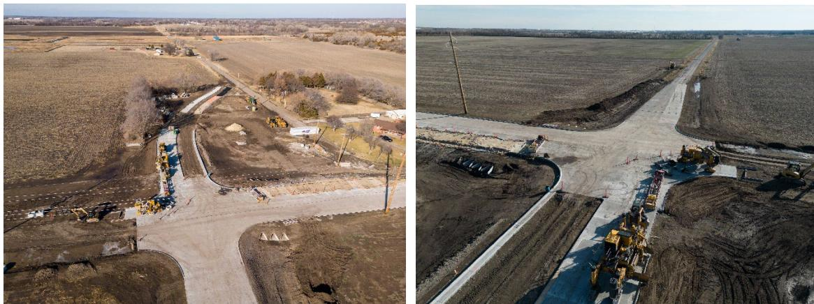
Here are 2 views of the Ford/Seneca intersection. Notice the progress on the re-alignment area, turn lanes and grading on the south/east part of the intersection.
